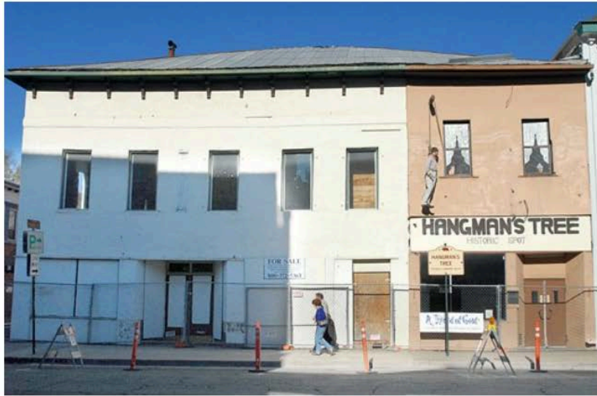
Herrick Building before restoration.
